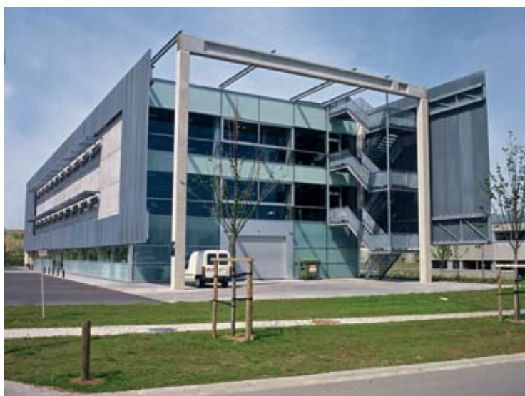
4 Transics, Ieper – arch. Buro Il, Roeselaere
