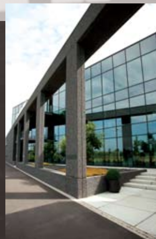
CET, Gullegem – E&L architects, Kortrijk
